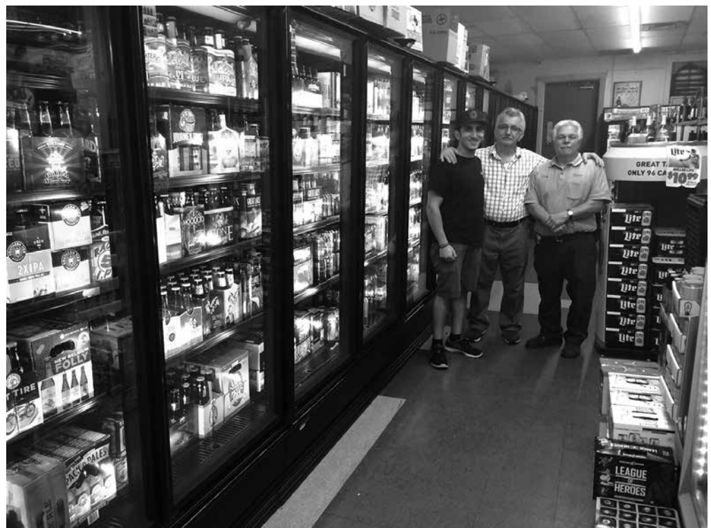
Charlie Eadeh, middle, with his son Michael, left, are joined by the installer at their newly commissioned, state-of-the-art cooler!
