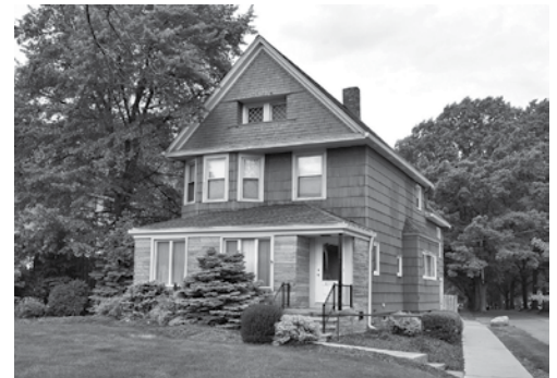
Frederick Barthelman built this house on Lorain Avenue around 1920. It was later moved to Rocky River Drive where it is now the office of orthodontist Casey L. O'Connor.
