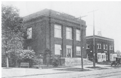
West Park City Hall (center) was only two years old when this photo was taken in 1916. West Park Fire Department at right. Courtesy of Raymond J. Kinkelaar.
