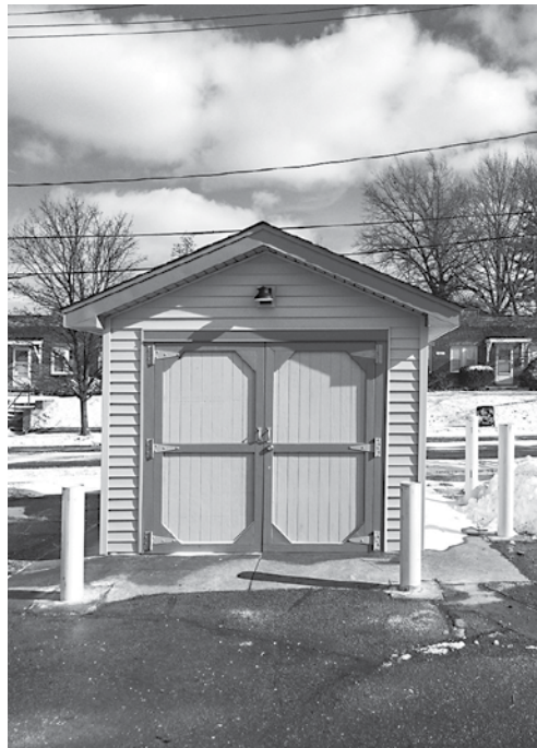
A new shed stands ready for Kamm's Corners Farmers Market and maintenance equipment.
