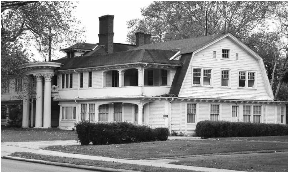
The shrine originally stood in the yard here – at the Marquard Mansion on Warren Road. Photo November 1, 2017.
