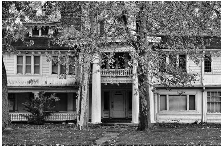
Marquard House, front entrance on Warren Road. Photo November 2017.
