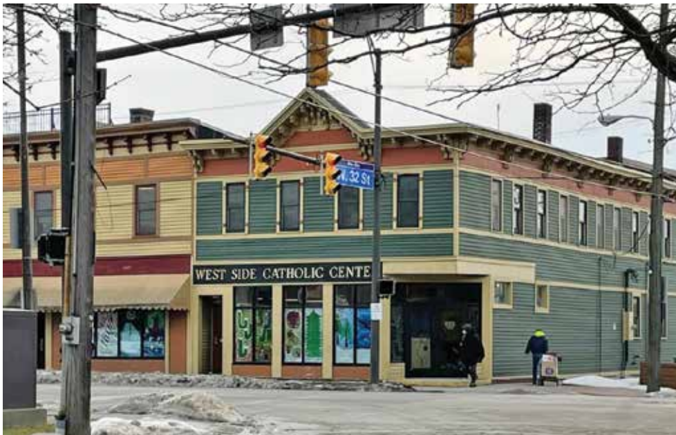
The West Side Catholic Center
