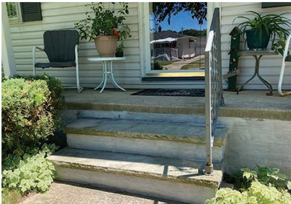
A step repair before and after
